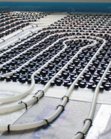
Visualisation of the AIRCONOMY® system modules installed in the floor.
